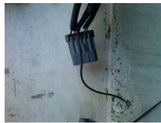
Re-wired connector with extra earth wire for high beam
